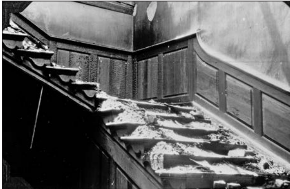
Charred panel section, Bassett Hall, ca. 1753, AF-1.22.1. The panel was removed from the damaged main stair after the 1930 fire.
