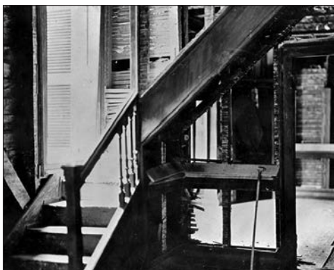
Servants' Stair Baluster, Bassett Hall, ca. 1753, AF-1.22.7. The baluster and stair (still in place just after the fire) were removed during the subsequent restoration of the house.
