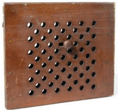
Ventilator from Mount Lebanon North Family dwelling house. Journalist Hepworth Dixon wrote in 1867, “The Shakers, who have no doctors among them, and smile at our Gentile ailments, take a close and scientific care of their ventilation.”
