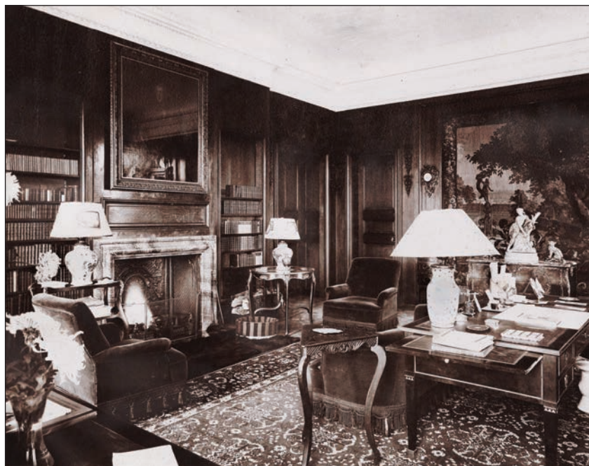
Southwest view of the library at the Mount
