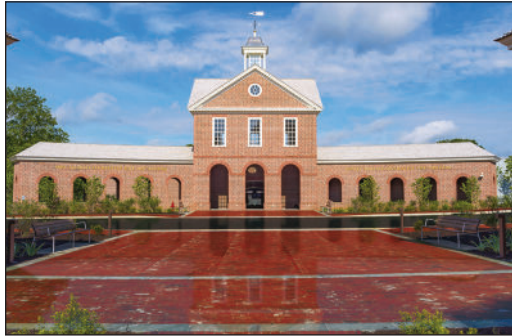
Figure 1: The Art Museums of Colonial Williamsburg front entrance. Colonial Williamsburg recently completed a 65,000 square foot expansion providing additional exhibition spaces and a dedicated entrance pavilion.
